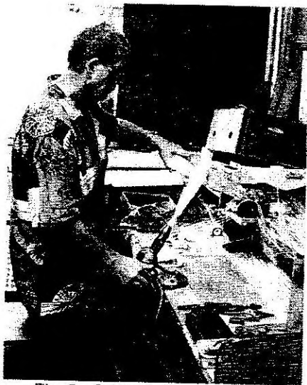
Fig. 2. Cutting tubing for bulbs.
